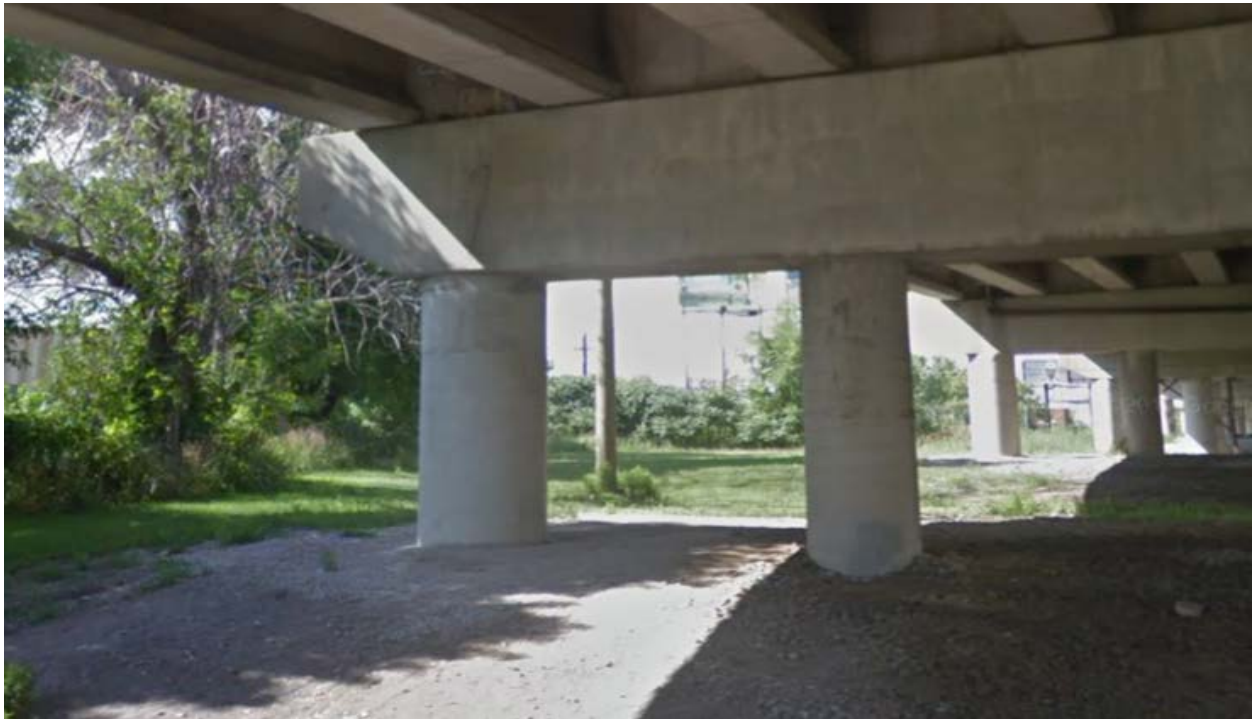
Above: Typical Column Repair completed in 2013.
