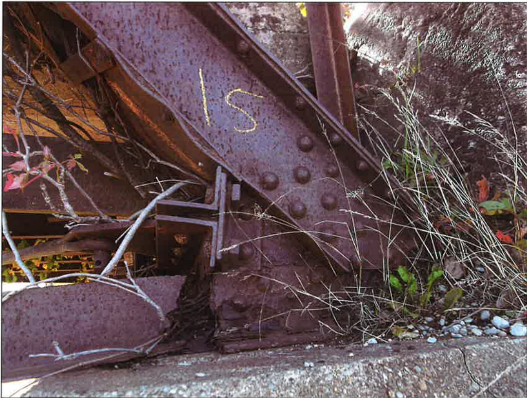
Bearing Seat at Northwest Corner of Bridge
