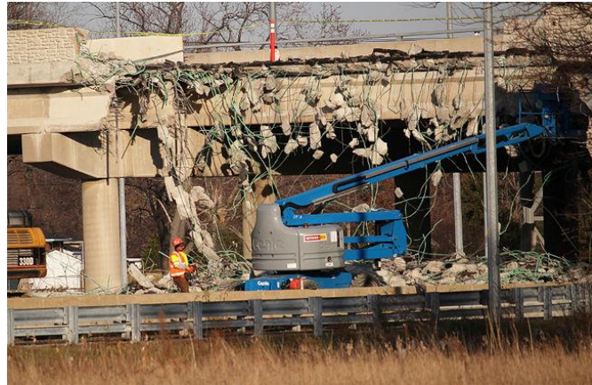
Figure 2-1: Repairs to Hwy 402 Bridge from Oversize Vehicle
