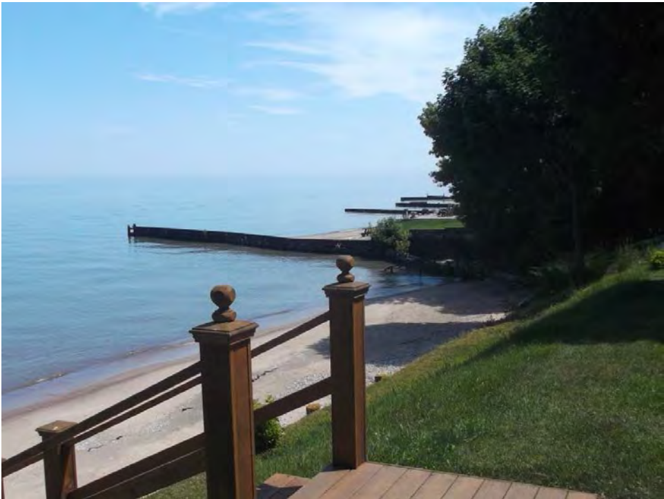
Photo 6: Steel sheet pile groyne to east of subject property
