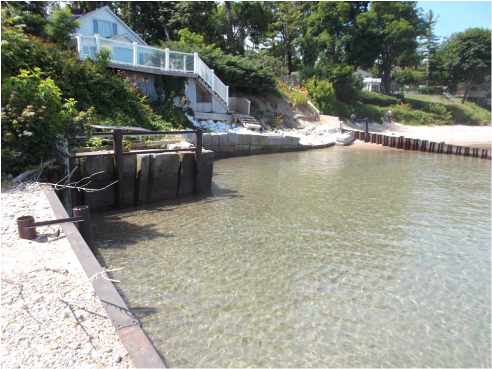
Photo 7: Shore protection works on property to the east
