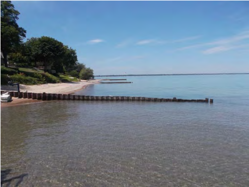
Photo 5: Steel sheet pile groyne system to west of subject property
