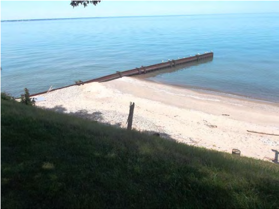
Photo 4: Steel sheet pile groyne to west of subject property
