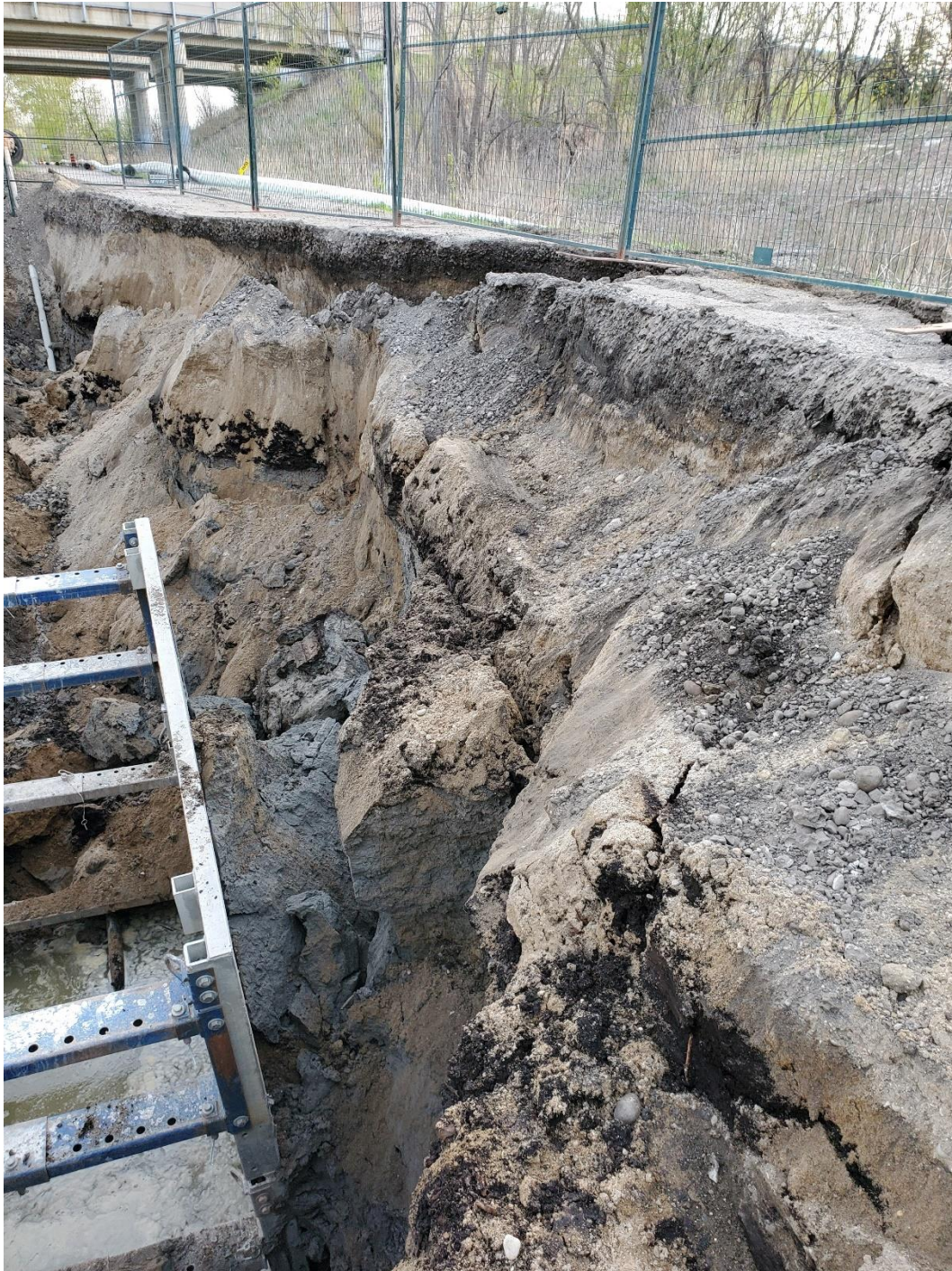
Image: Fencing surrounding excavation site.
