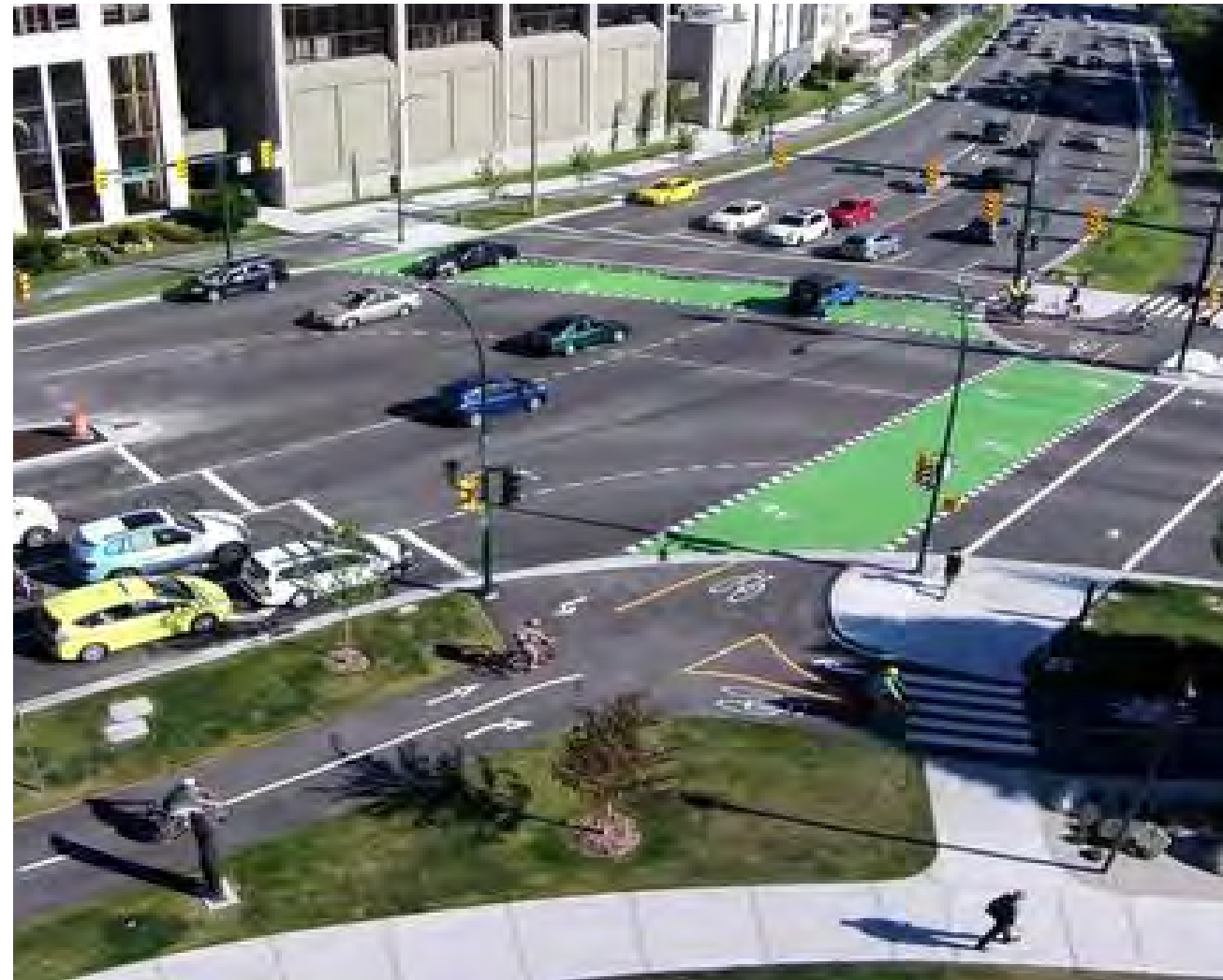
Figure 49: Protected Intersection in Vancouver
