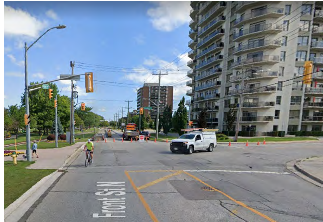
Figure 43: Front Street and London Road, Google StreetView. The intersection has no pedestrian phase which forces cyclists to go down their bikes to press the pedestrian button. Curb extensions at the intersection could also reduce crosswalk distance.
