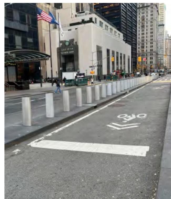
Figure 2: Segregated unidirectional bike lane in NYC, USA
