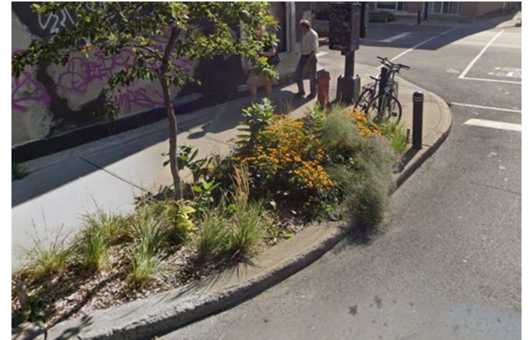
Figure 31 : Bump-out in Montreal.
