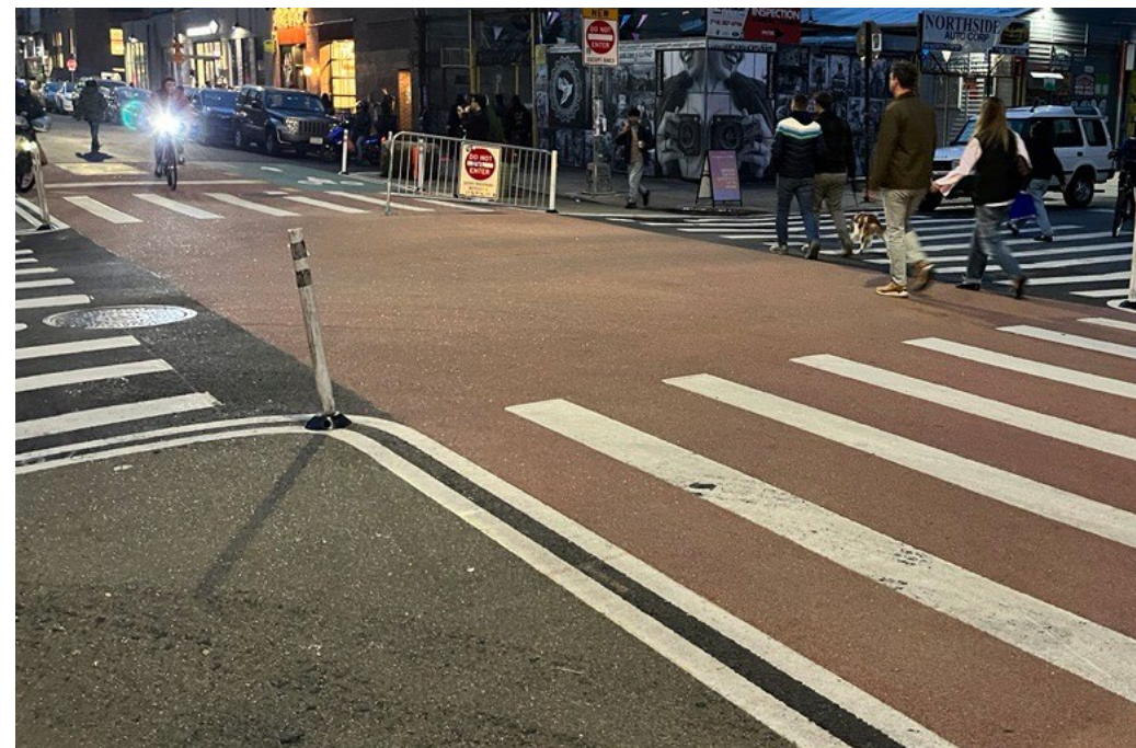
Figure 40 : Raised crossing and extension of sidewalk at pedestrian crossing in New York, USA.
