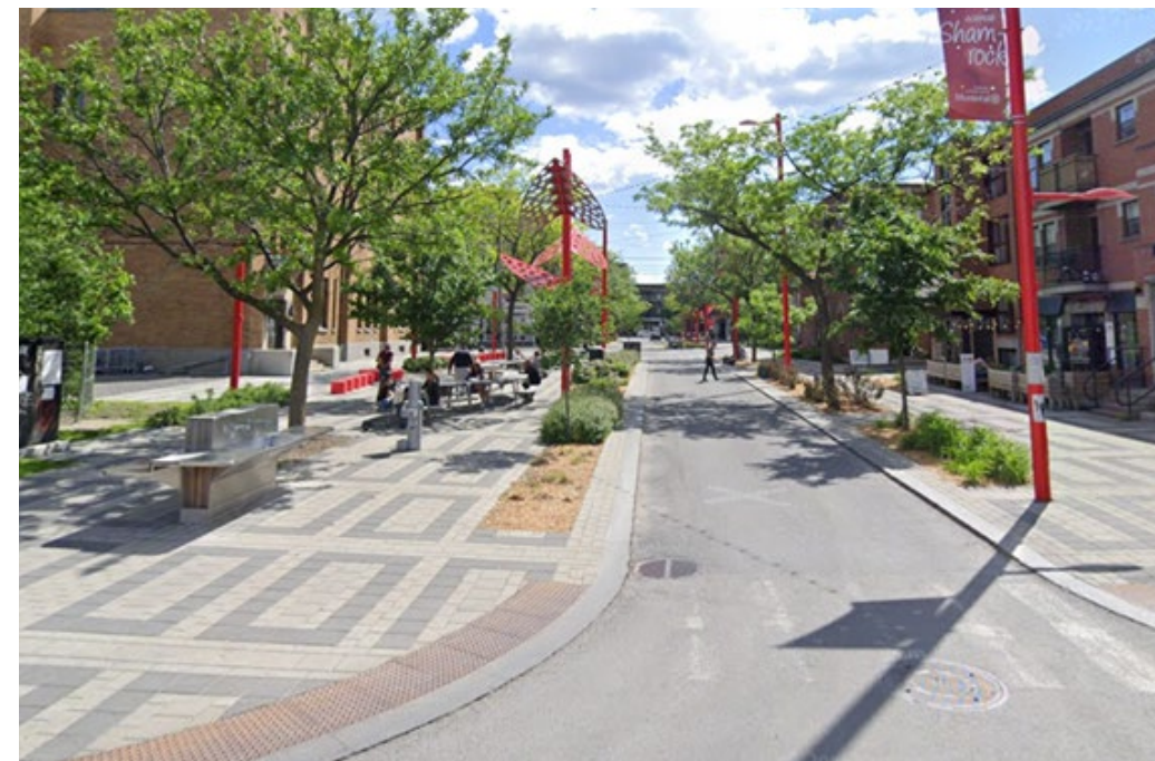
Figure 32 : Complete Street in Montreal.
