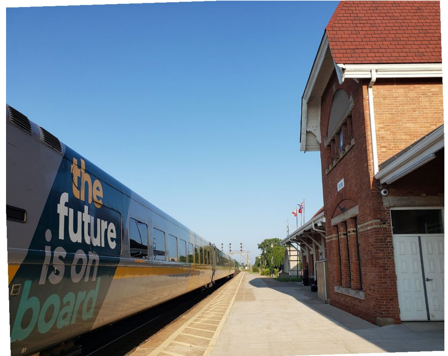
Figure 45 : Sarnia VIA Rail Station
