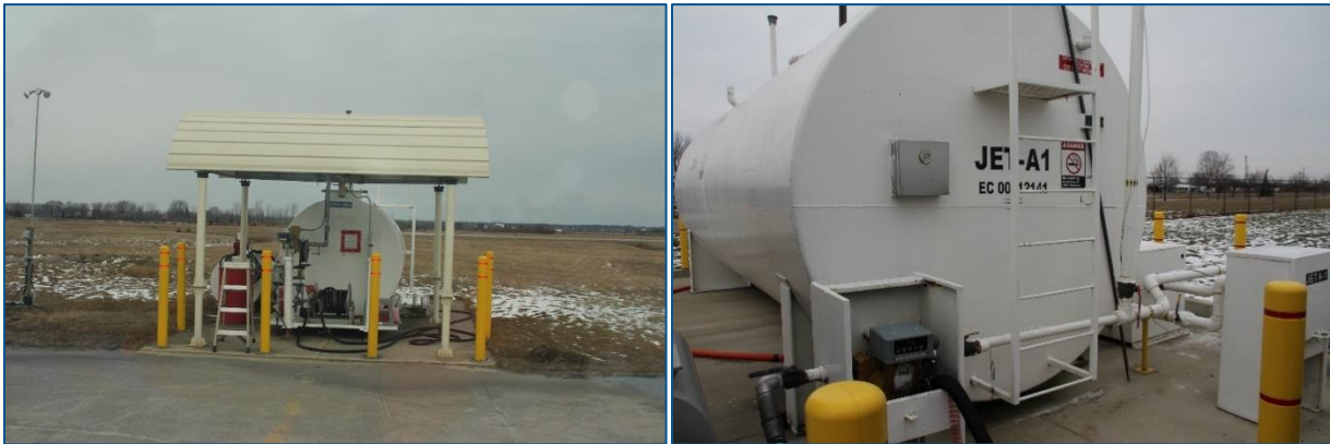
Avgas (left) and jet fuel (right) systems
