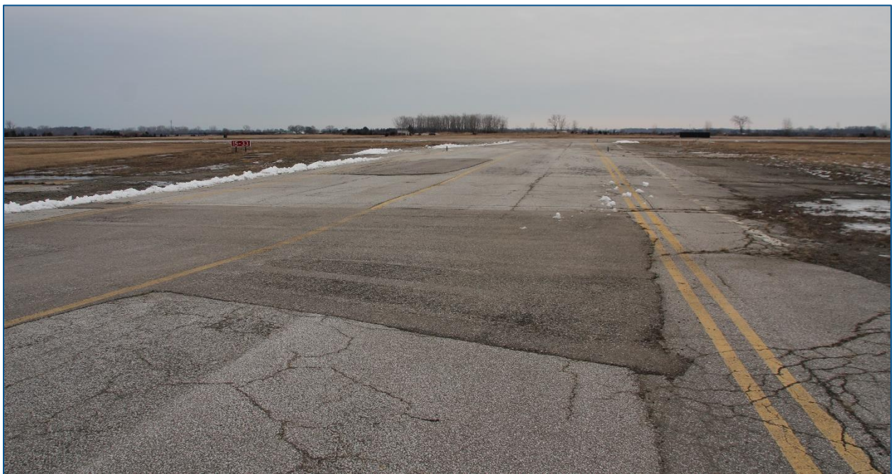
Taxiway A pavement condition
