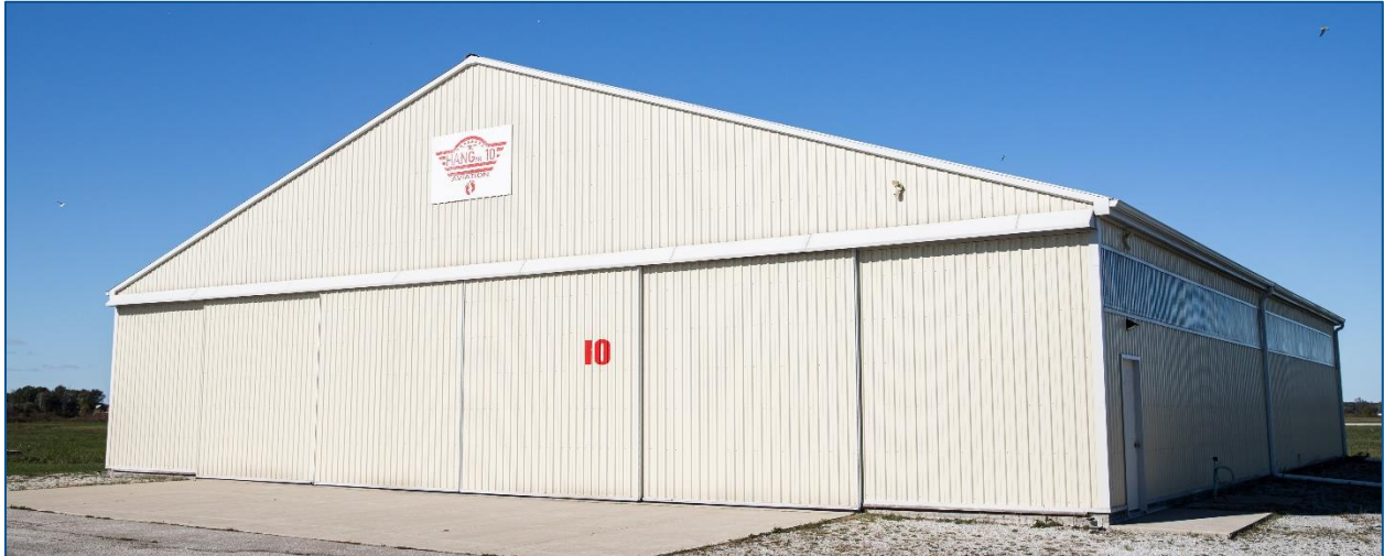
Private General Aviation Hangar
