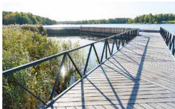
Example of floating boardwalk.
