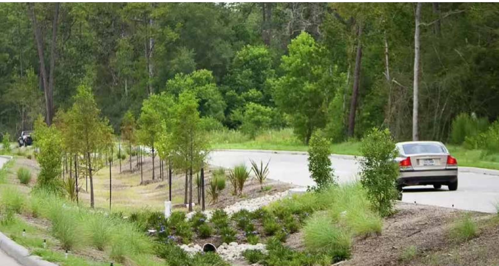
Example of vehicular road with integrated stormwater management.
