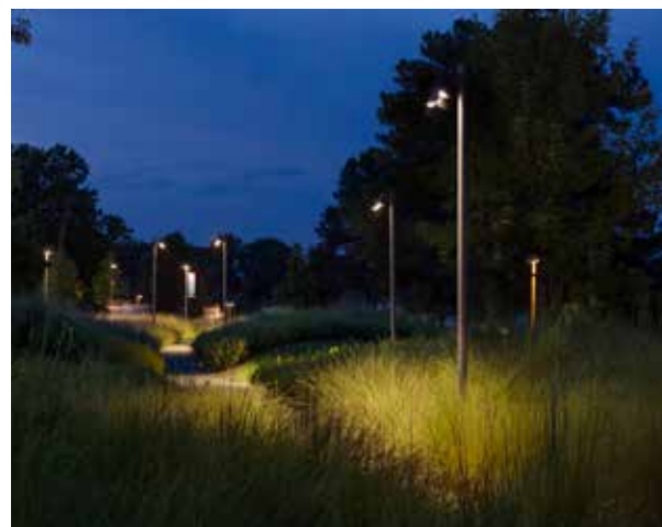
Example of shielded, down facing accent lighting.
